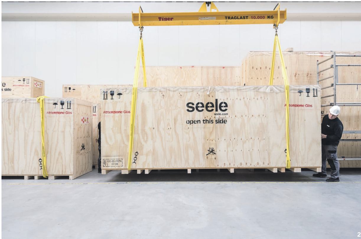
2+3 Safe transport: Every façade element had its own bespoke transport packaging, e.g. a wooden box, so that it could be safely transported.
