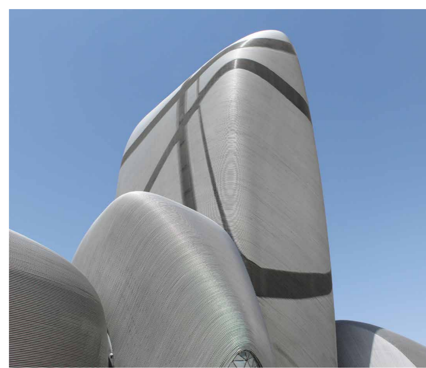
↑ Rohrfassade des King Abdulaziz Center for World Culture in Dhahran, Saudi-Arabien
