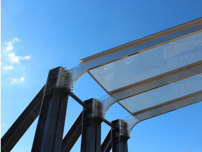
Mock-up at the testing grounds in Gersthofen. ©seele
