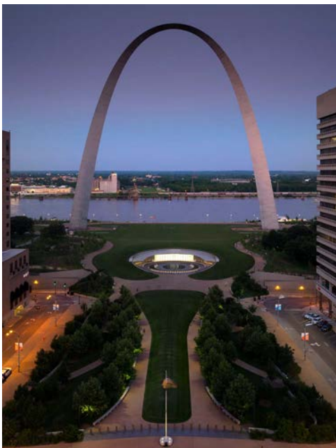
The new layout of Gateway Arch Park. ©Nic Lehoux
