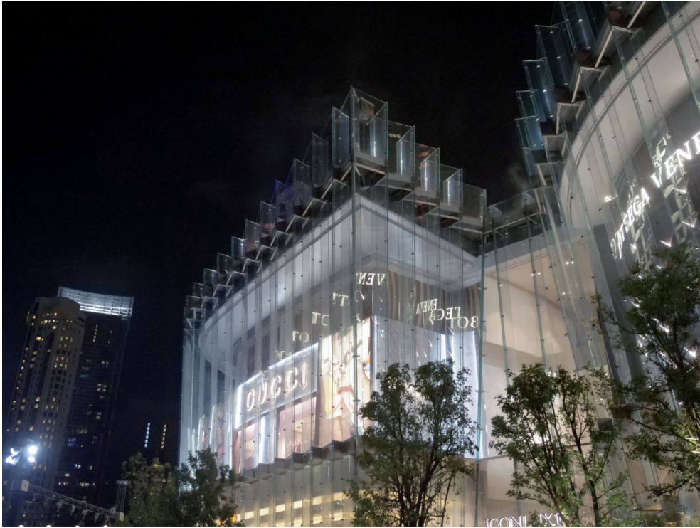
The pleated arrangement of the façade panes and glass fins alludes to the Thai leaf folding art of "Baisri". © seele
