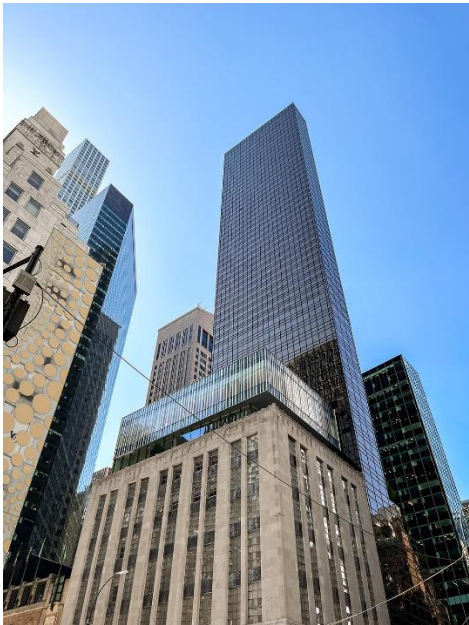
For the newly designed flagship store of Tiffany & Co., which is now known as “The Landmark”, seele realised the extension on levels 8 to 10. © seele
