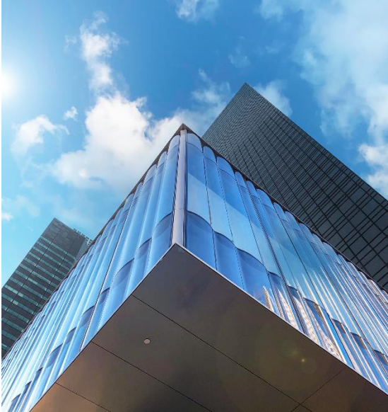
View of the installed wavy façade. © seele
