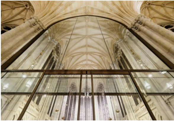
Internal façade of St. Patrick's Cathedral, New York, with surrounding brass cladding © Stephan Wurster
